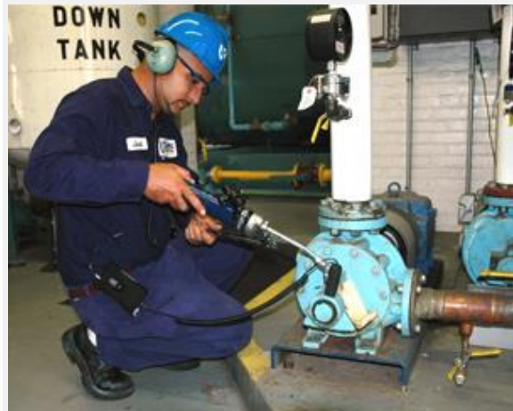
Figure 6. When applying grease to bearing on a pump, apply a little at a time and observe the meter for a dB drop.
