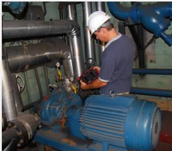
Figure 4. If used correctly, vibration analysis can give the maintenance and production team a heads-up on developing problems so that maintenance can be scheduled at the most convenient and cost-effective time.
